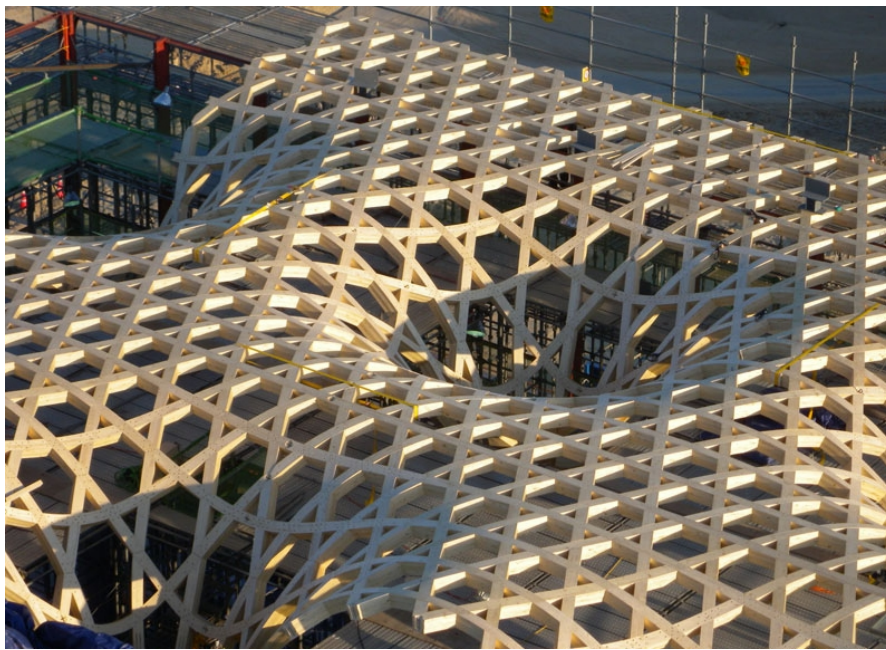
Figure 3.2: The roof structure of Yeosu Golf Club, South Korea, designed by Shigeru Ban, manufactured from timber using NC machining.
