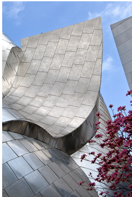
Figure 1.3: Details of the freeform exterior surface of the Walt Disney Concert Hall, which is realized using stainless steel panels. Photos by Renee Silverman and Richard Banks via Flickr.
